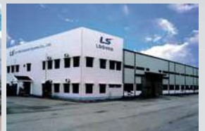
Hanoi factory (Vietnam) MV/LV switchgear, Mold TR
